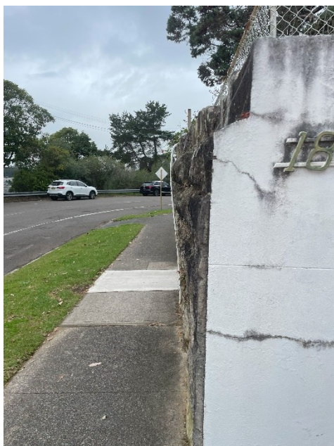
Plates 1 and 2 - View looking south showing bulge within No. 183 Greenwich Road front boundary retaining wall.
