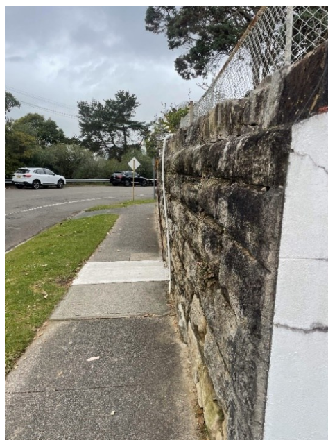
Plates 1 and 2 - View looking south showing bulge within No. 183 Greenwich Road front boundary retaining wall.
