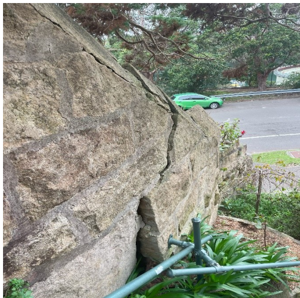
Plate 4 - Photograph looking East of failed retaining wall between No. 183 Greenwich Road and No. 4 Landenburg Place.
